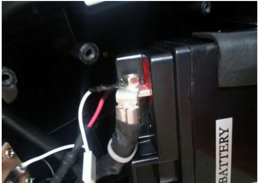
Fig. 159 - Securing the wire to the hot terminal of the battery
