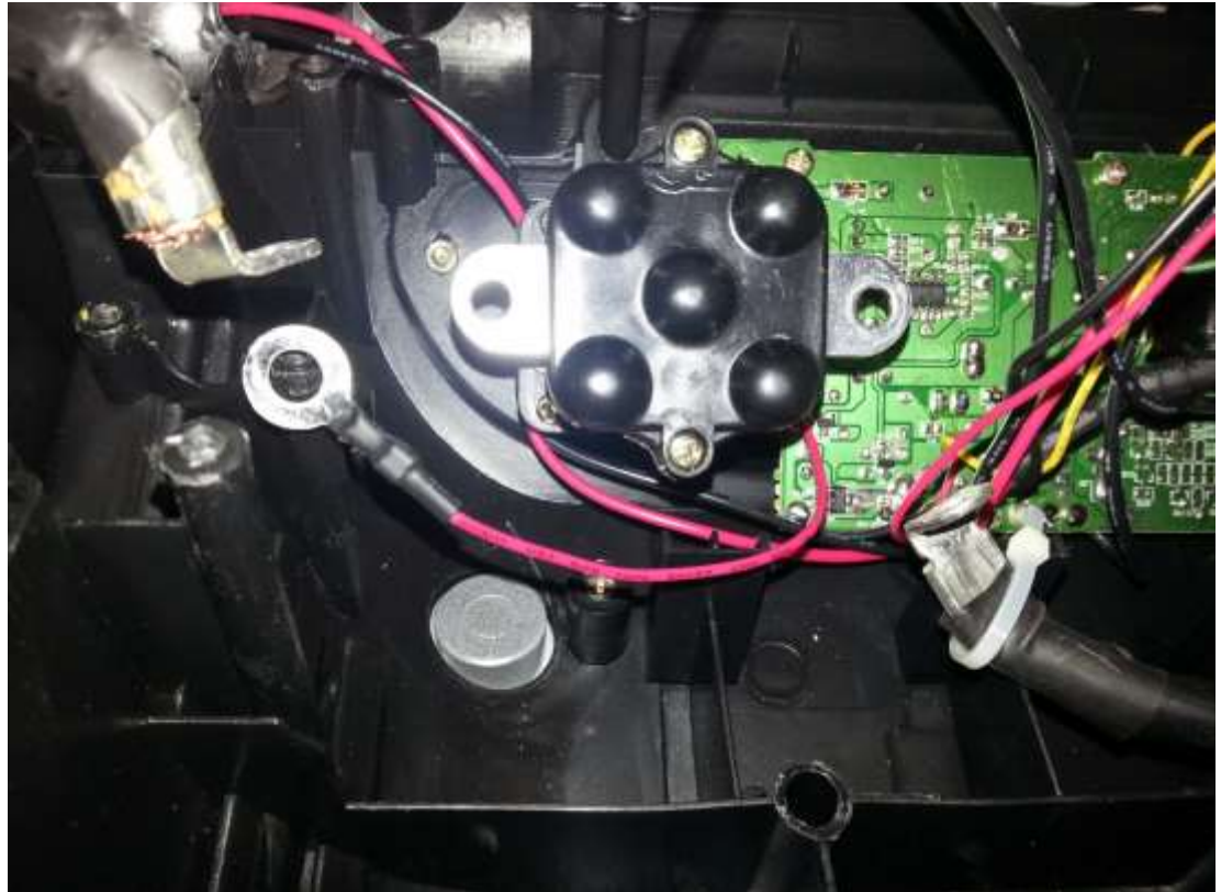
Fig. 154 - Preparing to attach the wires
