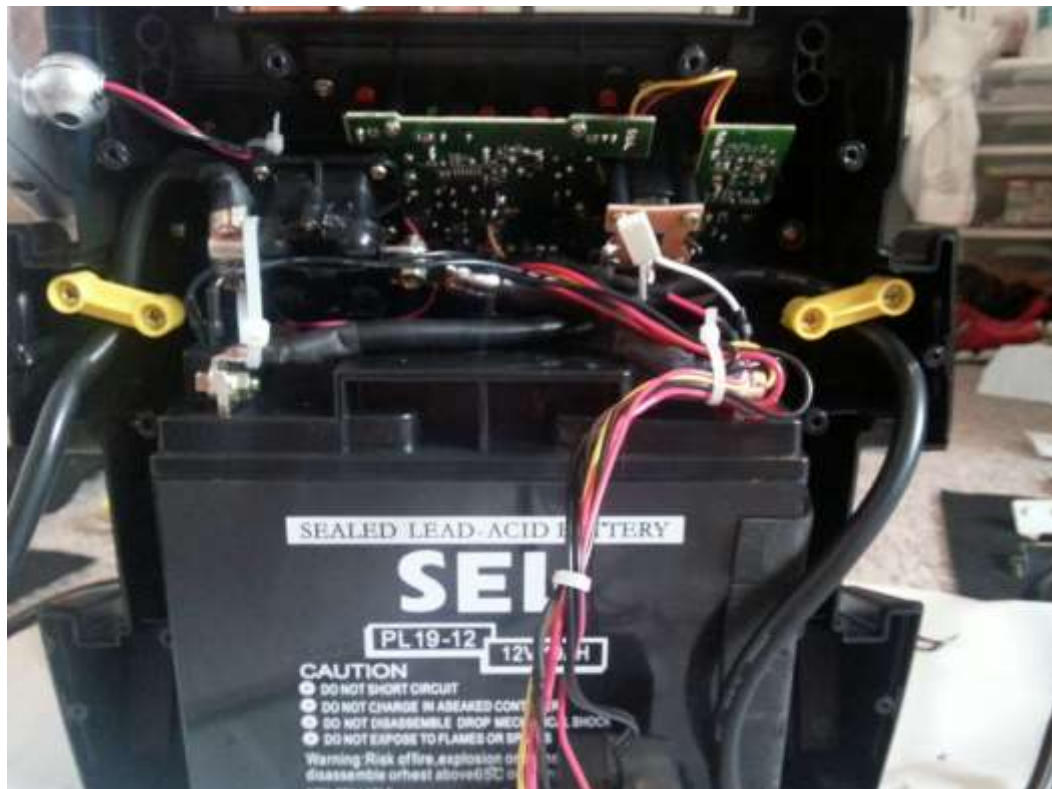
Fig. 162 - After securing the wire tie downs
