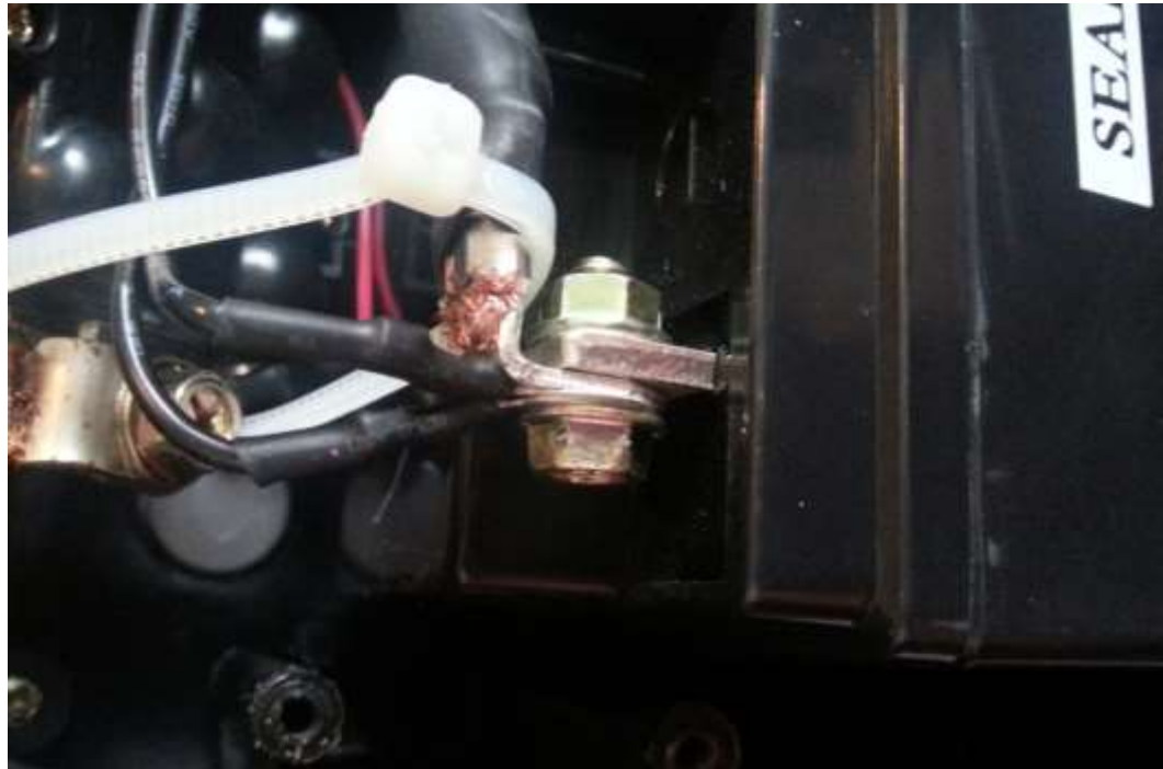
Fig. 157 - Attaching the wires to the ground terminal
